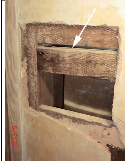
Old floor boards re-purposed as wall framing
