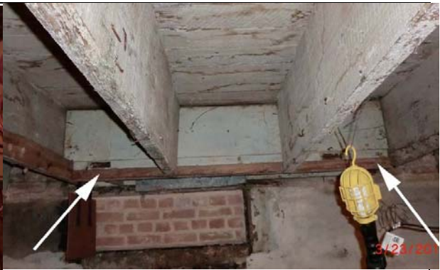
Old door jamb used as framing around an AC floor register
