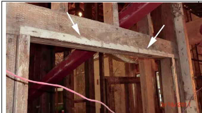
Former adjustable kitchen shelf brackets re-purposed as furring
