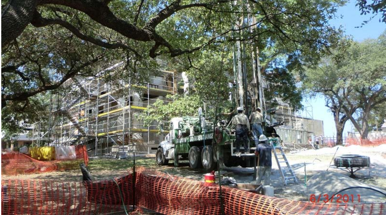
One of 45 wells being drilled on the Mansion grounds, to provide a heat sink and heat source for the home's new HVAC system
