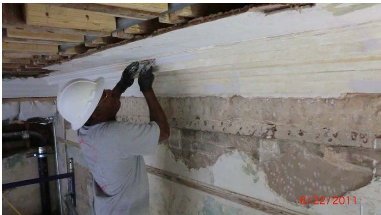
Artisan repairing plaster cornice
