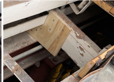
IMG_8986 pavilion rafter repair.JPG
