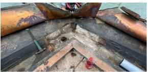
The 1949 and 1992 copper roofing is being removed and recycled by a facility selected based on highest price offered. All copper roofing not retained by the State is being recycled; there is no direct sale to the public planned as a reclaimed material.
