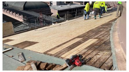
1/4" plywood underlayment will be placed on top of the historic wood decking to provide a smooth, consistent surface for the copper to lay on, without creating any condensation issues in the deck or clearances issues around any curbs. This will also absorb the impact of hail, minimizing dents in the copper.
