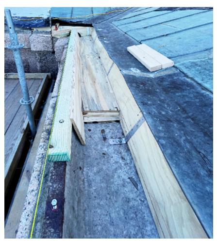
Gutter carpentry is underway, being built into the gutter carved into the top block of granite.
