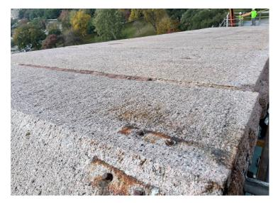
The south pediment will soon have its top joints sealed with lead tees to prevent water from entering these "skyward-facing" joints. This is particularly important to prevent damage from freeze-thaw cycles, and to protect the iron anchors that tie the masonry together deep in the wall.
