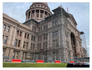
The south wing has been fully scaffolded. The north side of the east wing has been scaffolded, and now that we are in session, the south side of the east wing will continue between the hours of 7 pm to 7 am. The scaffolding is light in appearance, because it only is intended to provide fall protection at the edges of the roof, and a platform for workers to reach the gutters.
