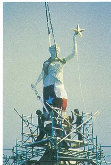
Above: CH-54A “skycrane” makes easy work of lowering the Goddess into place.
