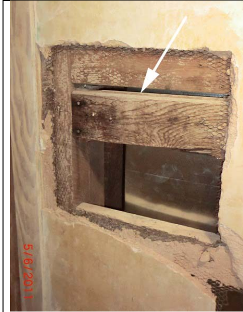
Old floor boards re-purposed as wall framing
