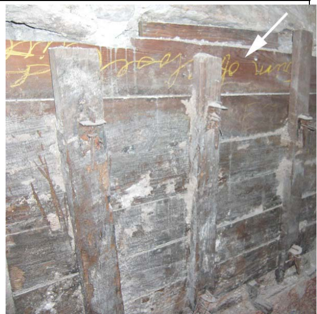
Old door trim re-purposed as formwork for basement walls
