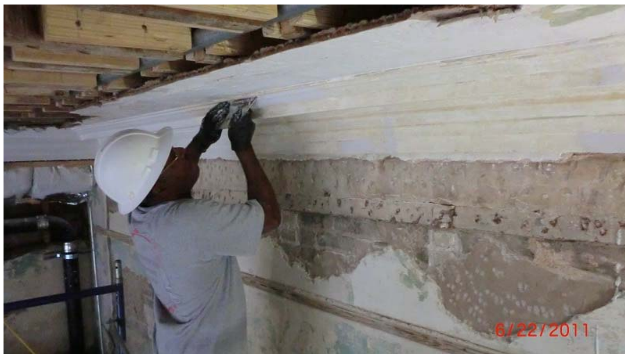
Artisan repairing plaster cornice
