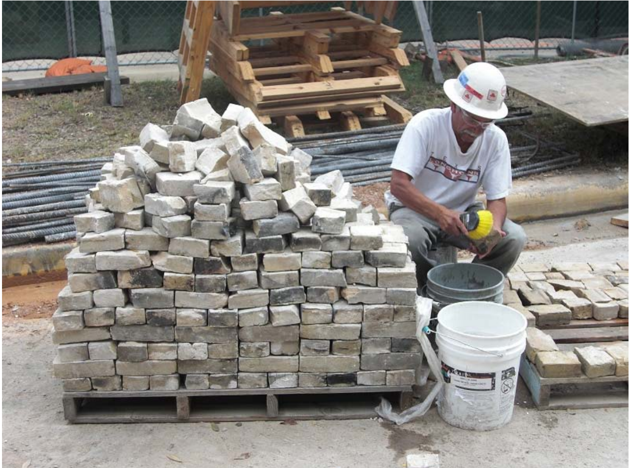
Worker cleaning salvaged bricks for re-use in the Mansion
