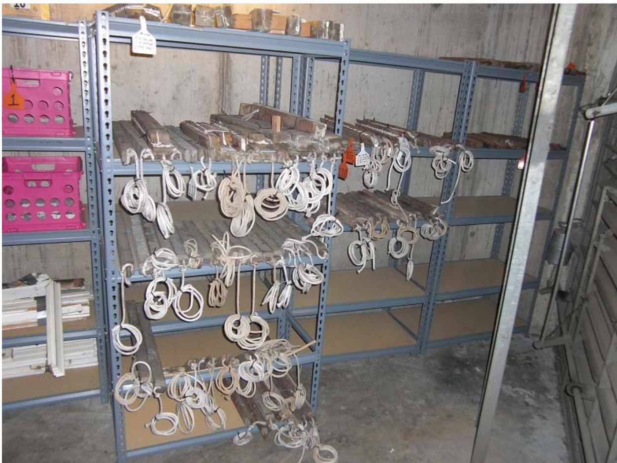
Original window weights awaiting re-placement with their respective windows
