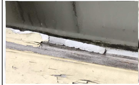
Paint Peeling and deterioration to exposed wood window elements.
