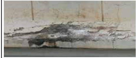
Stucco loss from water intrusion
