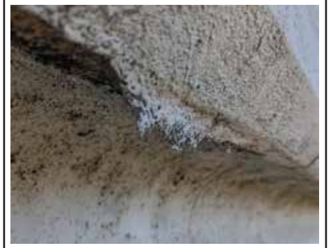
Paint staining and failure from water intrusion
