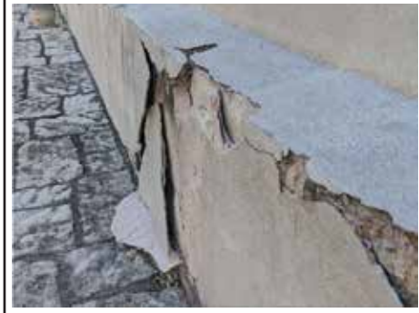
Stucco loss from water intrusion
