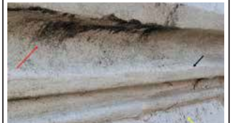
Paint staining and failure from water intrusion
