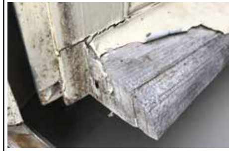
Paint Peeling and deterioration to exposed wood window elements.
